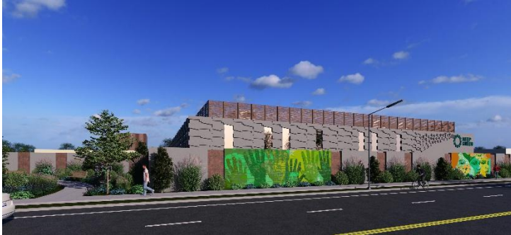
Proposed data center in Lansing, MI
