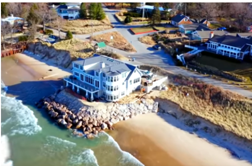
Armoring destroys the natural beach and accelerates erosion on neighboring properties.
