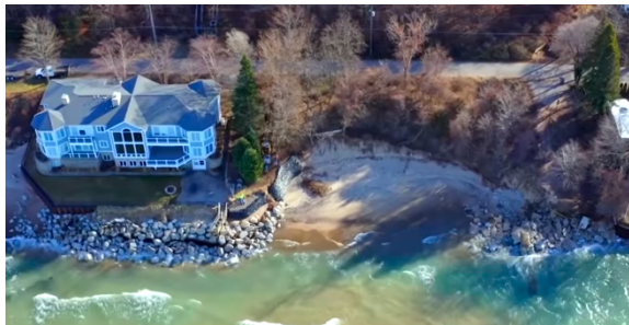
Armoring destroys the natural beach and accelerates erosion on neighboring properties.
