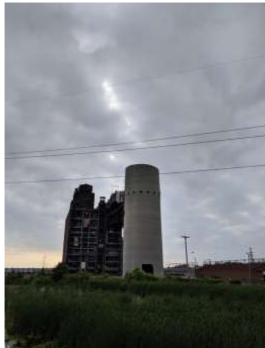
Figure 1: BC Cobb coal-fired power plant in Muskegon, Michigan, being dismantled, summer 2019. Photo by Sharlissa Moore.
